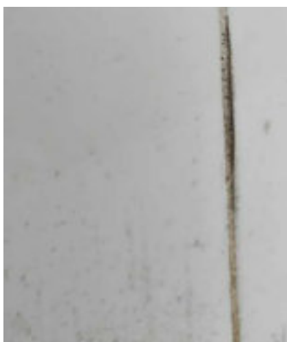
Image 17: Presence of water damage and mould in a property where the agent was unaware of the mould history
