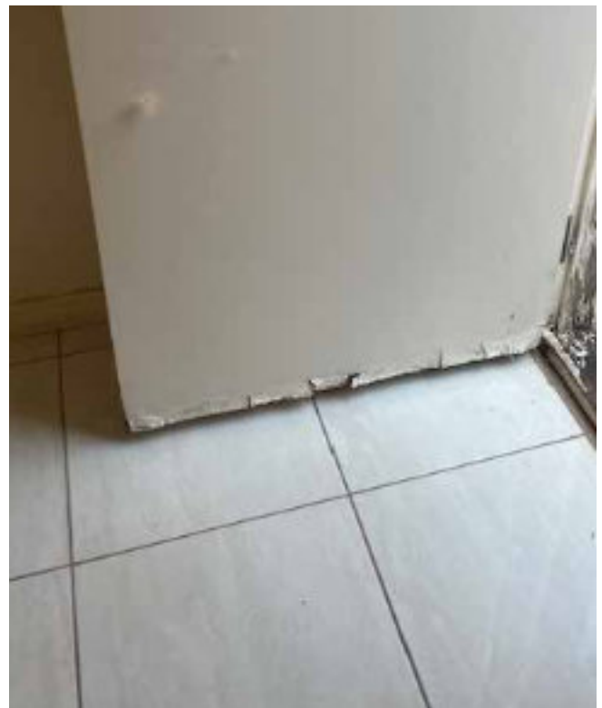
Images 26 and 27: Examples of poor maintenance- a broken light fitting and a damaged door
