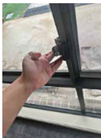
Image 3: broken window lock in Wyndham Vale, presenting a future security issue for a person renting the property.
